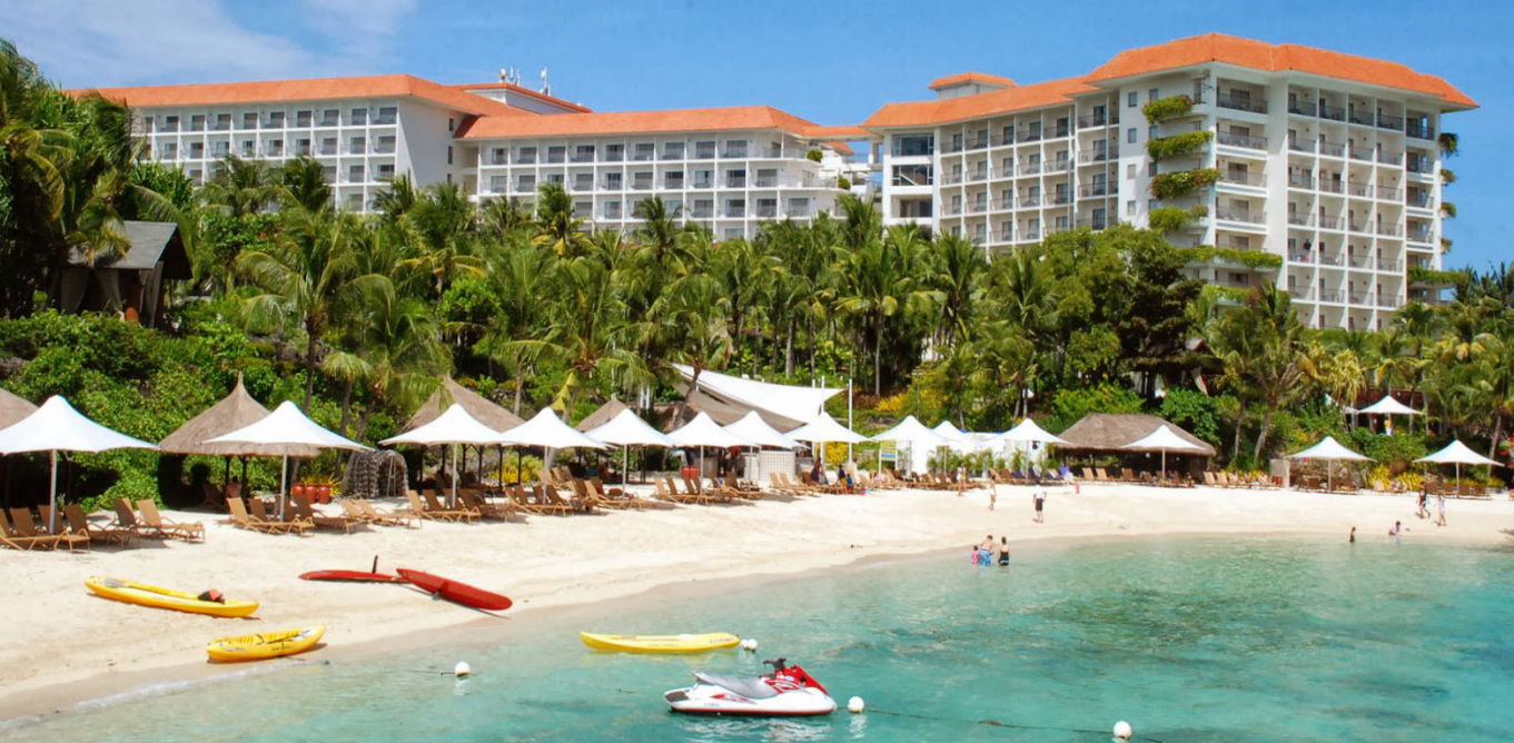
Image: Courtesy of H.S. Pow Construction and Development Corporation
